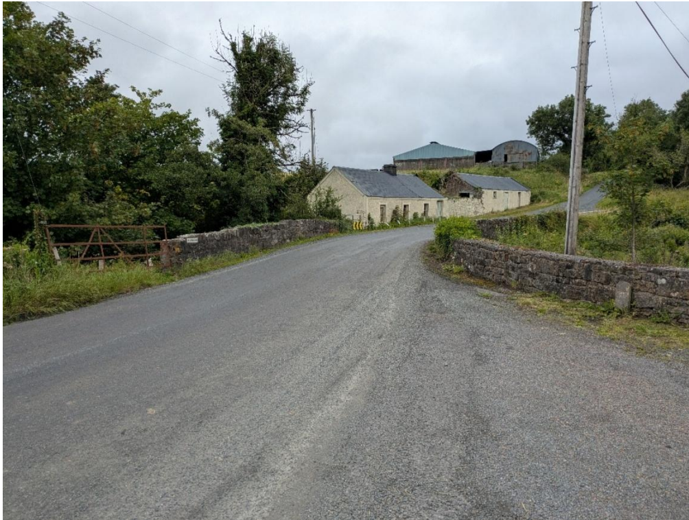
Plate 14-37 Bellanagare Bridge (CH69), facing northeast
