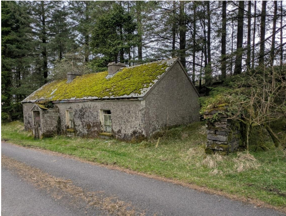
Plate 14-19 Location of CH16, facing west
