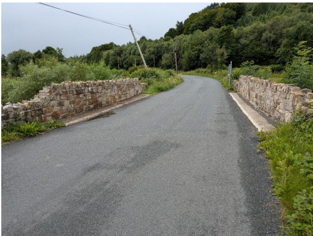
Plate 14-32 Bridge CH67, facing southwest
