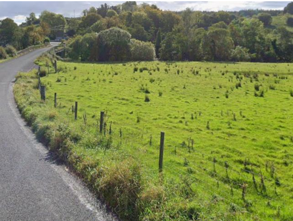
Plate 14-34 Section of the proposed grid connection that passes through greenfield, facing southeast
