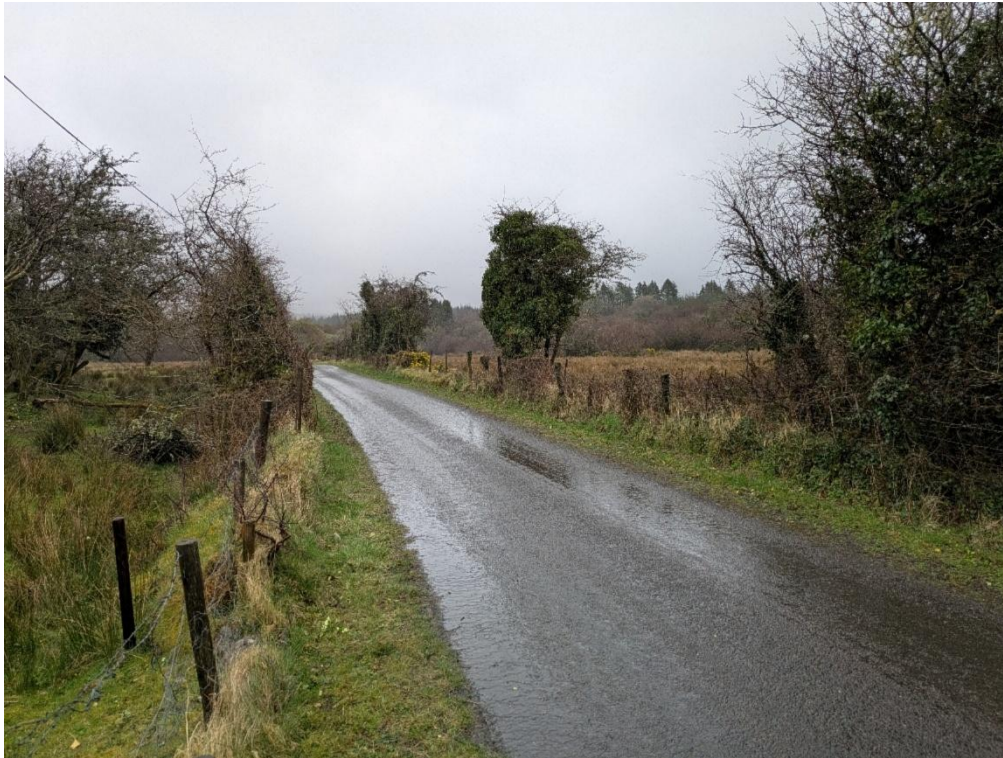
Plate 14-31 Location of proposed grid connection passing through ZoN of AH85, facing northeast
