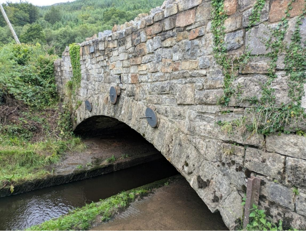
Plate 14-33 Bridge CH67, facing southwest
