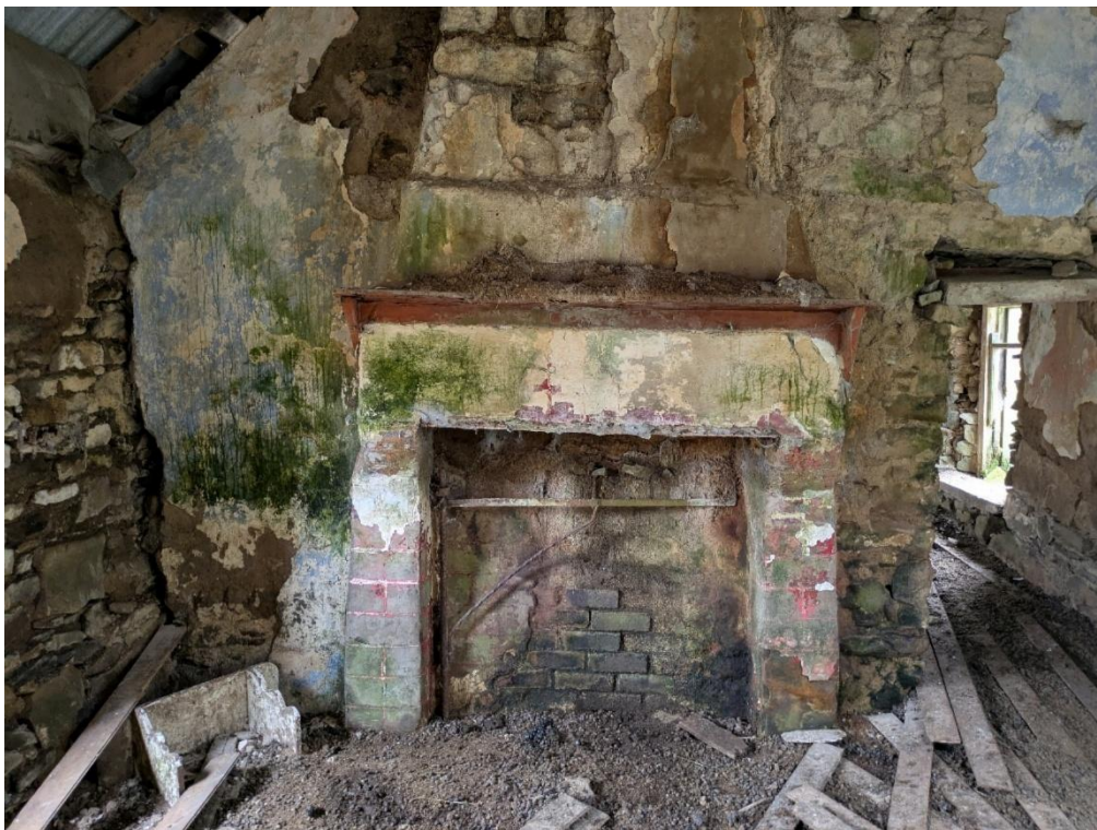
Plate 14-28 Interior of CH18, showing fireplace and fire crane, facing east
